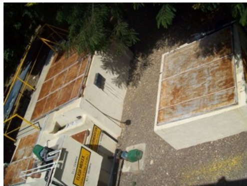
Effluent Treatment Plant
